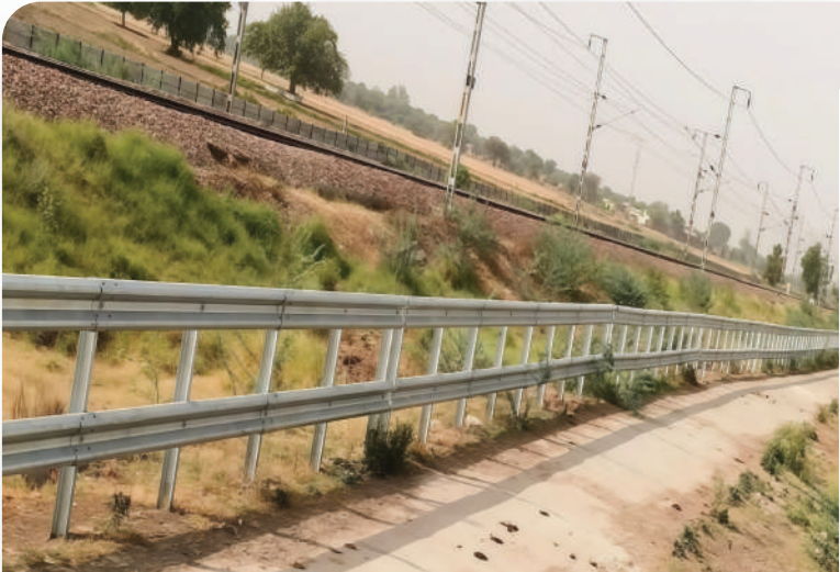
W / Thrie Beam Crash Barrier for Highways and Railways
